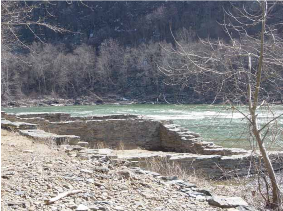
Figure 2: Historic structure losing ground to Shenandoah River. One of many examples of historic structures and features in danger of being washed downstream by the Potomac and Shenandoah Rivers at Harpers Ferry National Historical Park. Periodic, seasonal floods cause severe river bank damage and change channel morphology. Photograph by Trista L. Thornberry-Ehrlich (Colorado State University).
