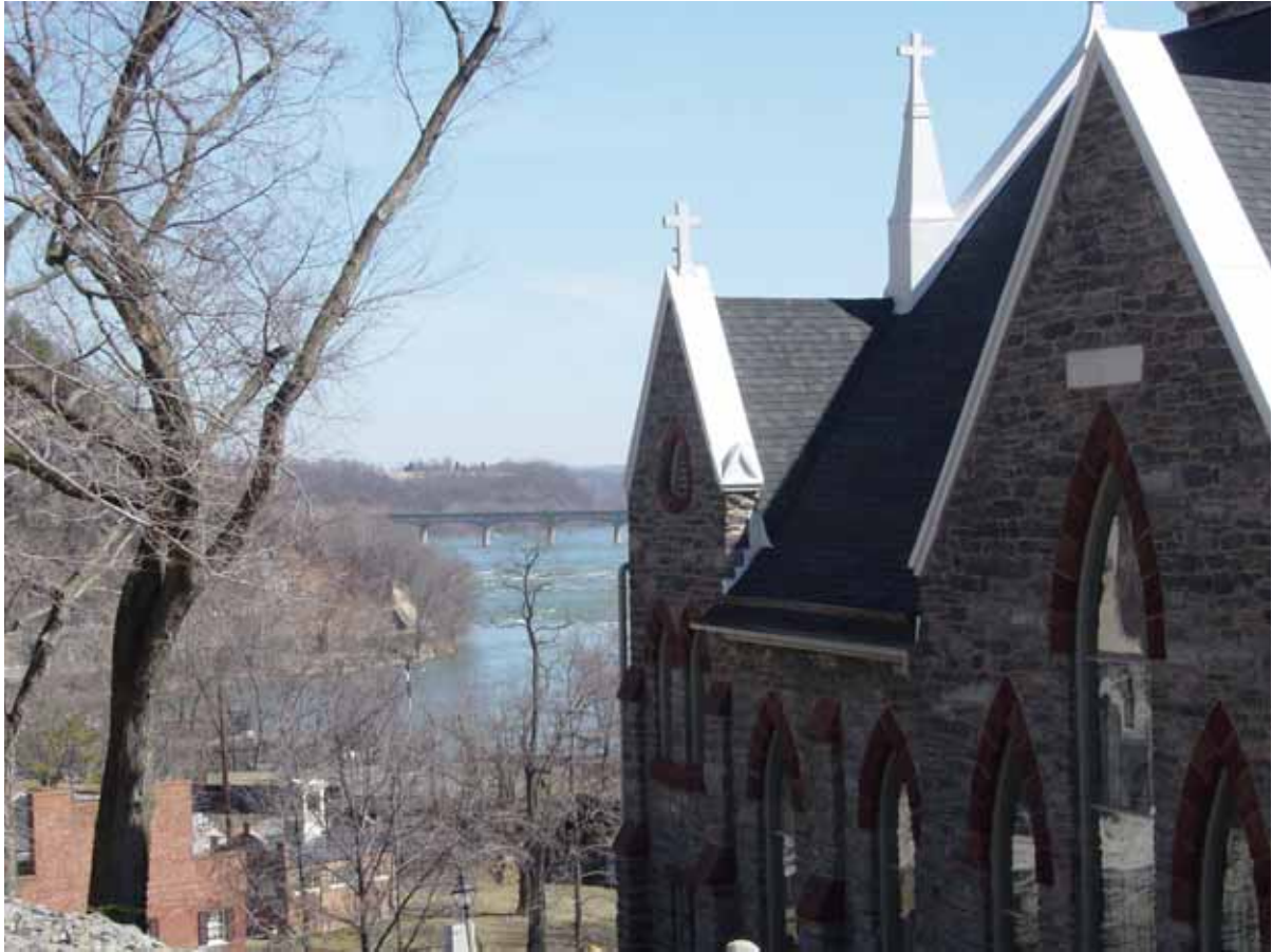
Figure 9: View of Harpers Ferry. Harpers Ferry sits on the slopes above the meeting of the Potomac and Shenandoah Rivers. This dynamic setting is inherently subject to flooding, river bank erosion, and channel morphology changes. The steep slopes within and above the town are prone to rockfall, slumping and sliding. This presents unique management issues when dealing with the preservation of the historic structures of the national historical park. Photograph by Trista L. Thornberry-Ehrlich (Colorado State University).
