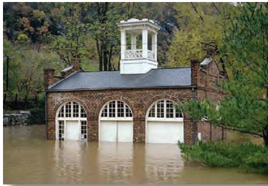
Flood waters at John Brown's Fort. Photo: NPS.
